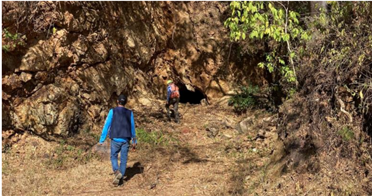
Figure 12-1 Stope as Found at the Location of the Napoleon Deposit (Center of the Picture)
